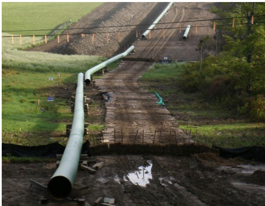
Empire Pipeline's Tioga County Extension Project. Source: Empire Pipeline
